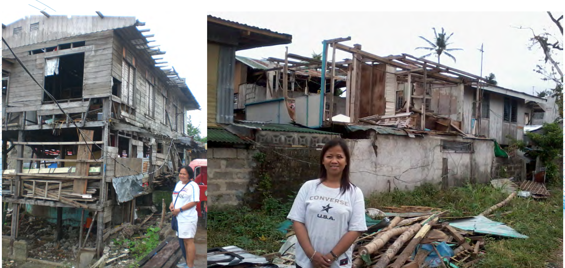
Destroyed houses of APCD's Emergency Support beneficiaries
