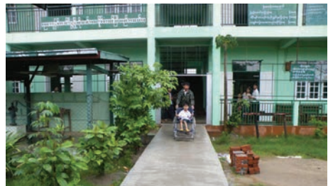
Building a ramp in school
