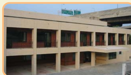
Training & Accommodation Building
