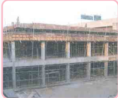
APCD's Training & Accommodation Building
