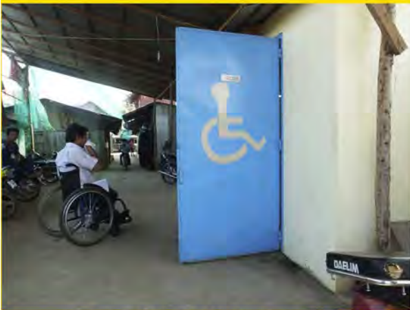
Accessible toilet at Phlou Thmey Market
