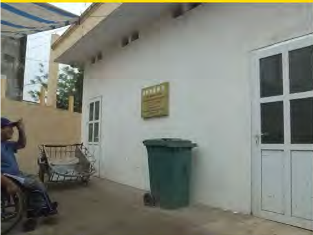
Accessible toilet at Nhong Market
