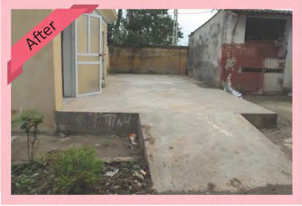
Market interior after modification
