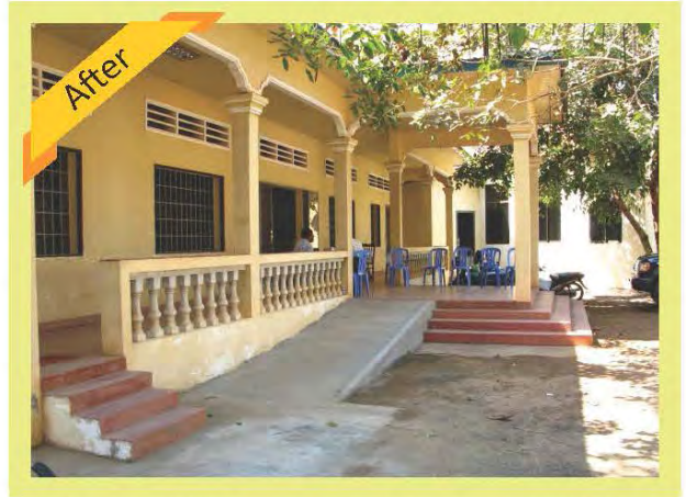
Ramp at the entrance of the Training Hall
