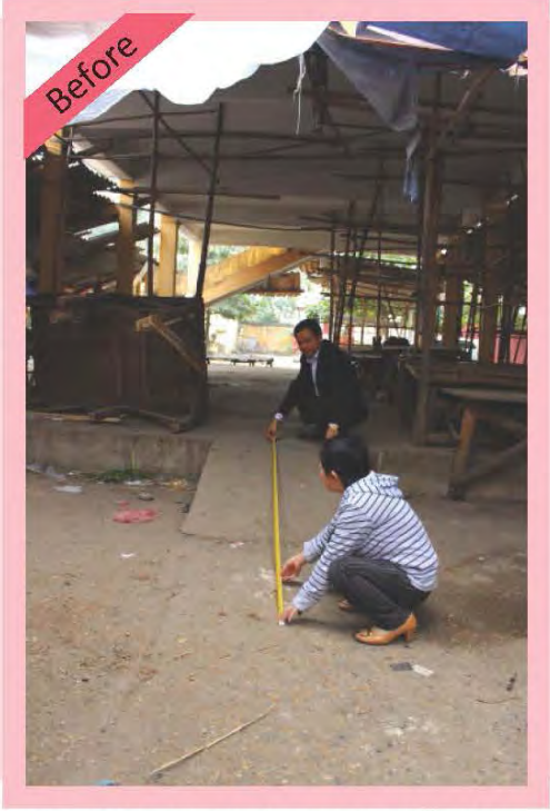
Market interior during modification
