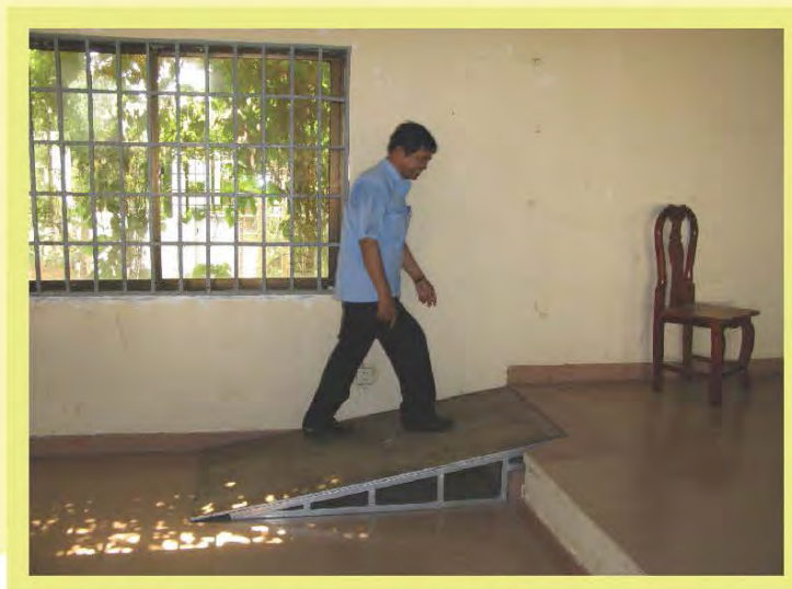
Ramp going to the stage inside the Training Hall
