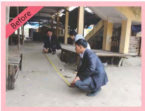
Market interior during modification
