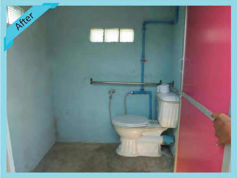
Interior of accessible toilet
