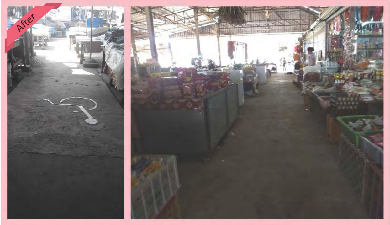
Accessible entrance and pathway in the market
