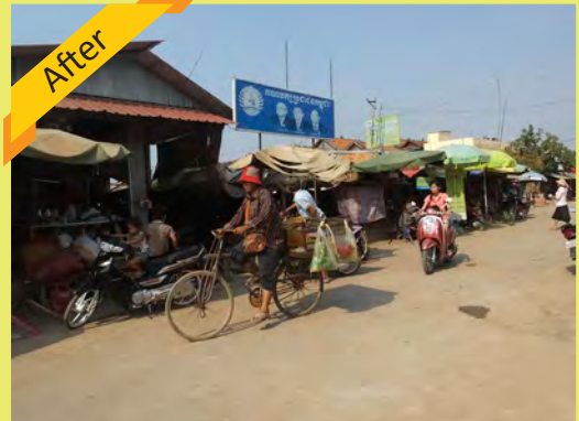
Paved road in front of the market
