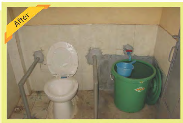
Toilet in the District Office Training Hall
