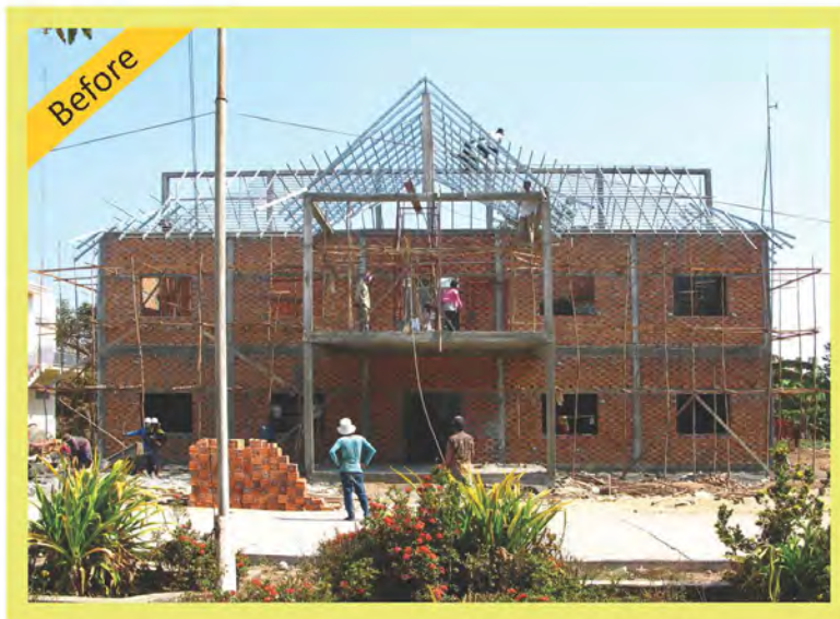
Workers during construction of District Office building
