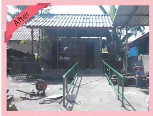
Ramp leading to the accessible toilet
