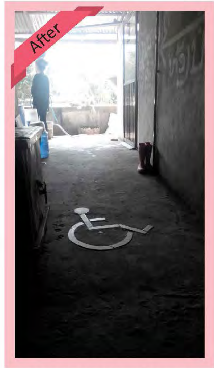
Accessible toilet with signage
