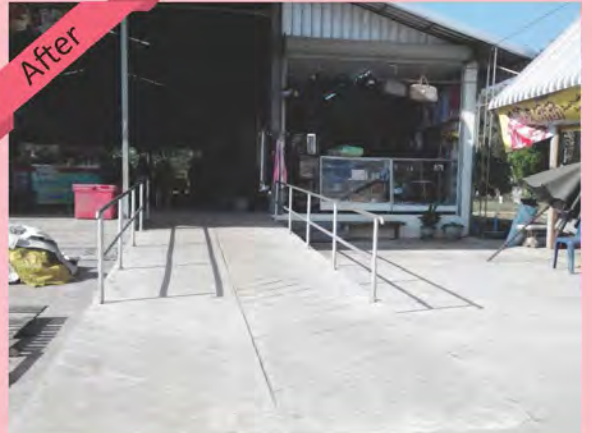
Accessible market entrance with grab bars
